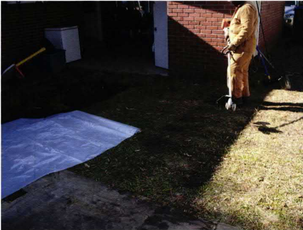
Picture 1: UST 609Dahlia-2 excavation is in progress. Technician is standing atop location of 609Dahlia-1.
